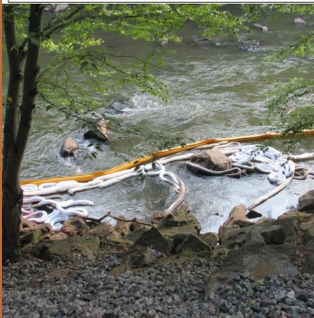
**Containment efforts directly below railroad bed to minimize ongoing seepage of fuel oil into the Stonycreek River. It is estimated that 1,500 gallons of fuel oil spilled from a railroad tanker car as a result of an accident with a truck at a railroad crossing.**
