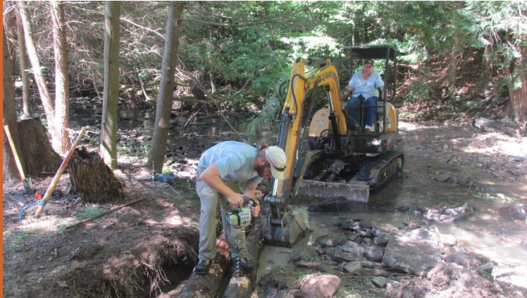
Greg Shustrick, Watershed Specialist for the Somerset Conservation District and Mountain Laurel Chapter Trout Unlimited member drills a hole in a log while backhoe operator and Trout Unlimited volunteer, Bill Conlin, holds it in place. Photo by Len Lichvar
