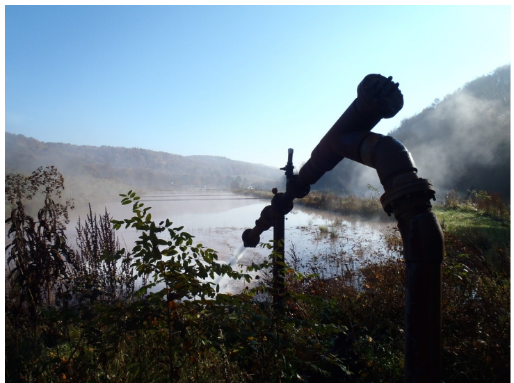
Spray nozzle at Lion Mining Company's Deep Mine Passive Treatment System on the Bens Creek
